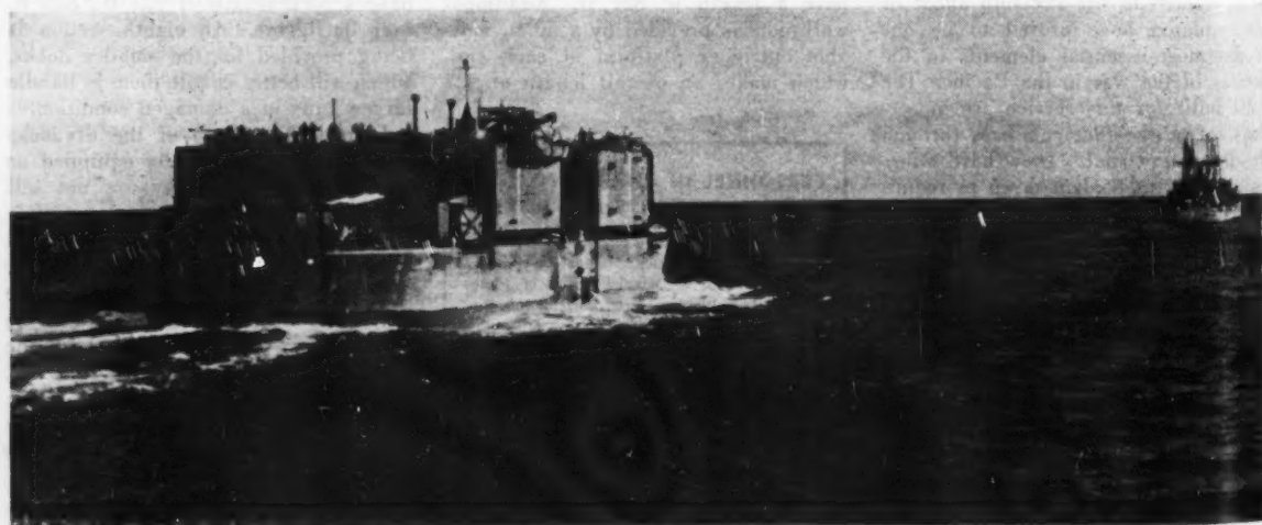
Sections of floating drydocks are towed at speeds of 10 mph. by a Liberty ship, which also carries a load of supplies for establishment of a new base.
